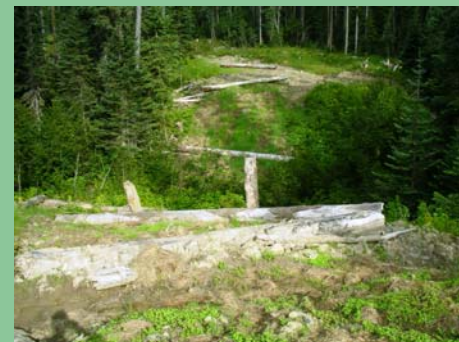
Stream crossings on in-block roads are generally only utilized for a year or two, after which they are removed. Cross ditches, re-vegetation and other erosion control measures (as depicted above) are then installed on higher risk sites to reduce the potential for sediment input into streams.
